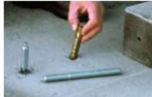
4. Remove any dust and small particles from the drill holes using a brush and compressed air. This will ensure perfect adhesion between the resin for the ground anchor and the concrete foundation.
