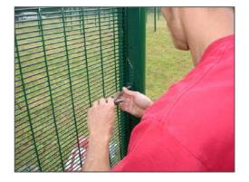
2. Fix the panel with 2 fixators to the first post
