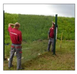
1. The panel should be bowed slightly to fit between the posts
