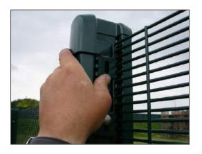
→ For the installation of flat Securifor on Bekafix Super posts, the installer can drill an <u>extra hole on top of the post</u> to be able to fix an extra fixator, to avoid folding the top of the panel
