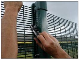
8. Align the panel and fix all the fixators on the second post (take away the middle fixator)
